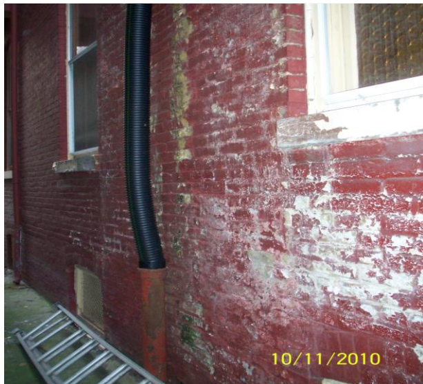
Connect the top and bottom of the pipe – a simple solution!
